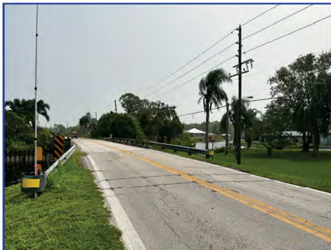
Catfish Creek Road bridge looking east.
