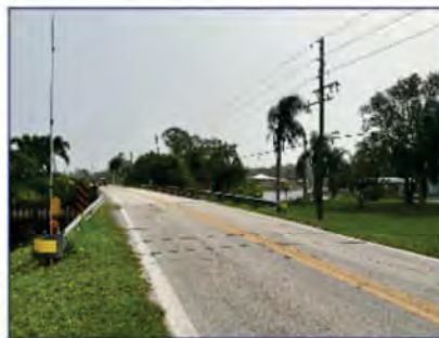
Catfish Creek Road bridge looking east.
