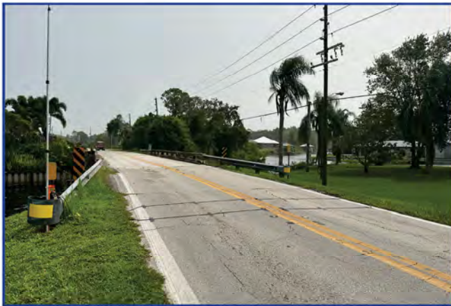
Catfish Creek Road bridge looking east.
