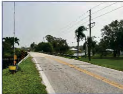
Catfish Creek Road bridge looking east.
